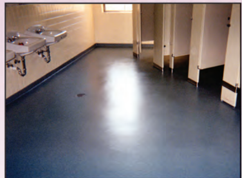
A slip-resistant finish combined with our Bio-Pruf additive makes cleaning and caring for your restrooms a breeze.
